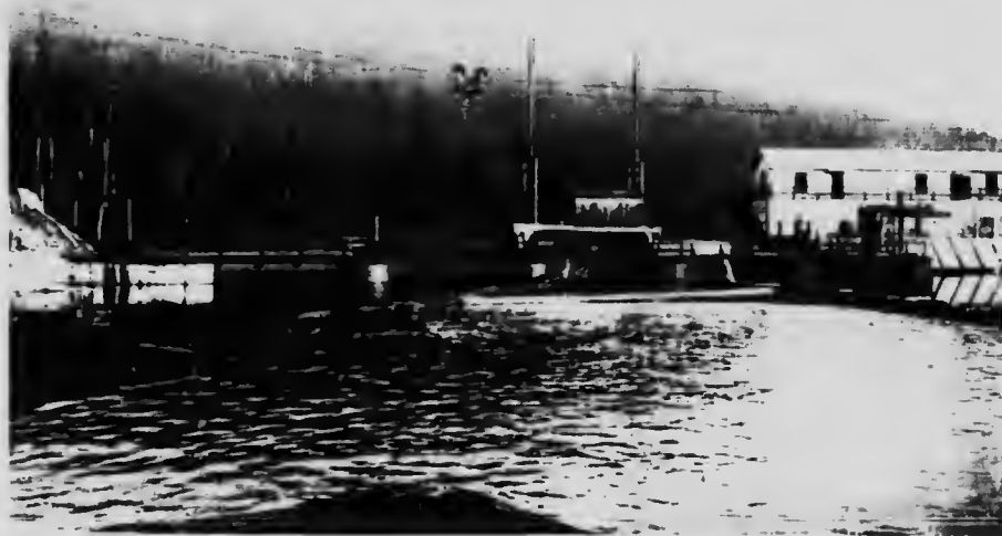
Stave Lake Development. Looking downstream above dam.
